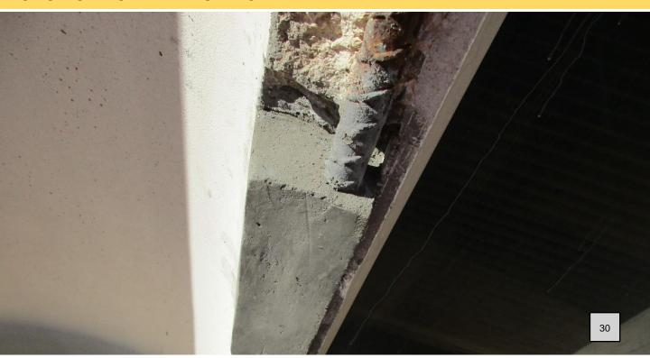
ANTICIPATED REPAIR: SPALLED CONCRETE REMOVED; TROWEL GI
