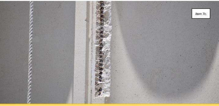
ABOVE: TYPICAL ANTICIPATED REPAIR WITH RUST FROM SHALLOW CAST REINFORCING BAR EXPANDING AND SPALLING CONCRETE AWAY FROM BAR.
