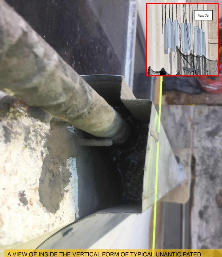
A VIEW OF INSIDE THE VERTICAL FORM OF TYPICAL UNANTICIPATED REPAIR WITH DETERIORATED CONCRETE BEHIND AS WELL AS IN FRONT OF THE CONCRETE REINFORCING BAR, FORCING A TOTAL RE-BUILD OF THE FIN USING FORMS TO RECONSTRUCT THE FIN USING POURABLE GRADE MATERIALS IN RELATIVELY LONG SECTIONS WHERE TROWEL 35 GRADE MATERIALS WERE NOT PRACTICAL
