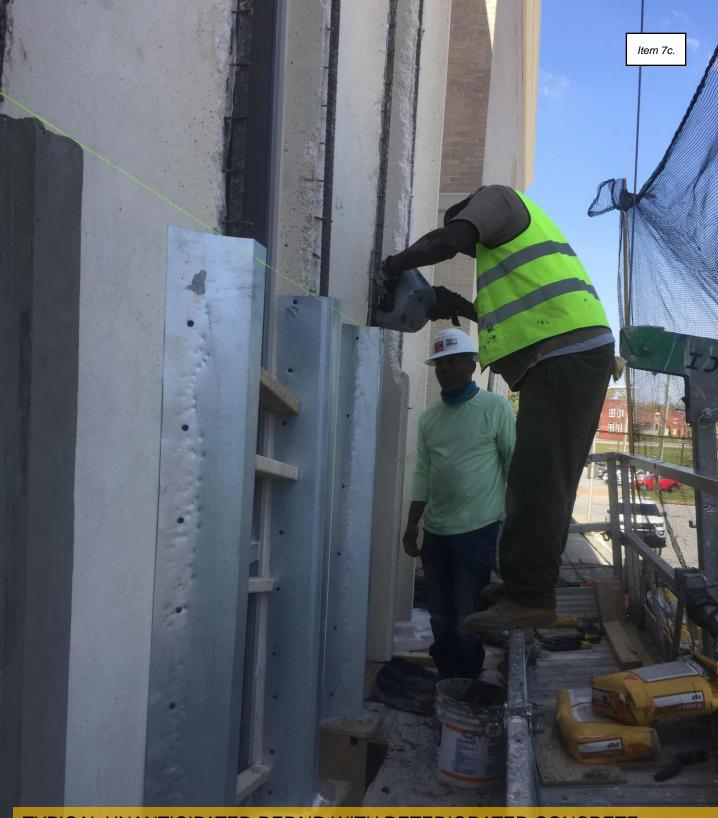
TYPICAL UNANTICIPATED REPAIR WITH DETERIORATED CONCRETE
